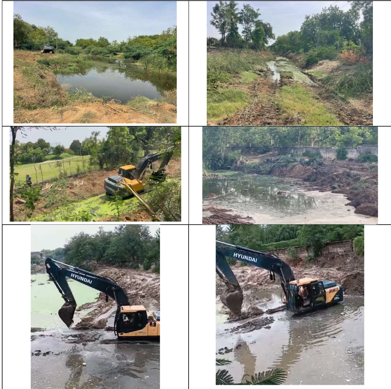
Figure 10.4: Photographs of de-silting operations
